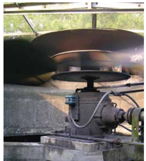
A typical conventional fan drive arrangement of a gearbox mounted under the fan.
